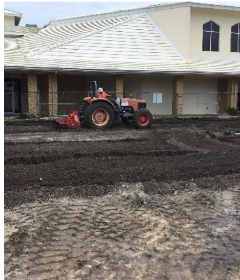
Mixing subbase in parking lot
