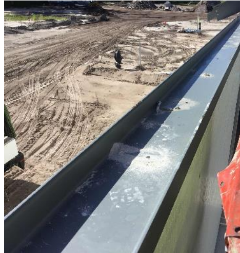
Spandrel Beam Installation
